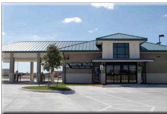
The new Austin Telco Federal Credit Union branch in Buda has a standing-seam metal roof.
